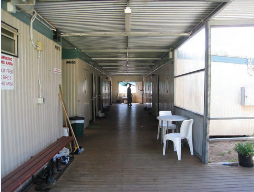
The extension to Unit 2 which was created with transportable units.
