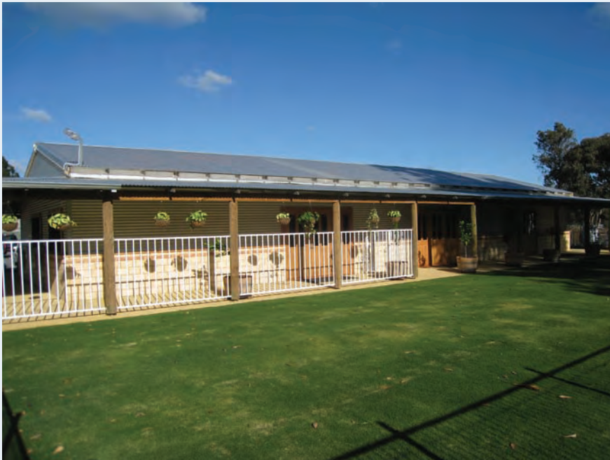
The new Shared Facilities Centre serves as the visitors' centre on the weekend and a staff training centre during the week. It is an impressive asset for the prison, and a significant achievement, having been built almost entirely by Karnet prisoners.
