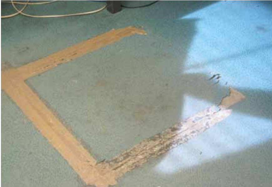
Carpet taped into place in Unit 1 pod.
