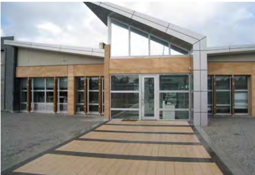
Back of the gatehouse.
