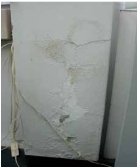
Mould on wall in ASPM's Office.
