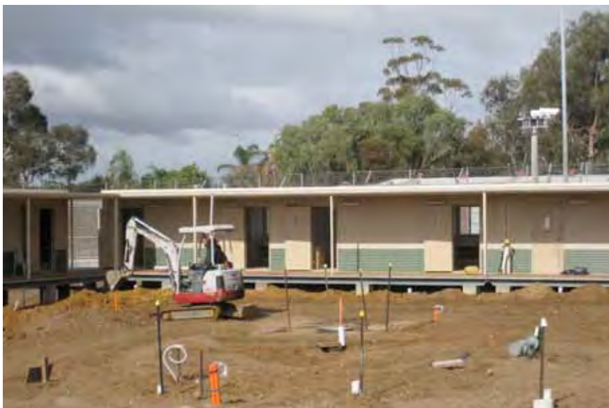
The demountables mid-installation.
