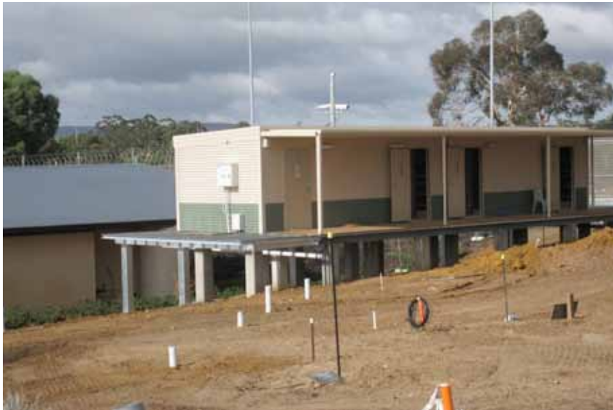
The demountables mid-installation.
