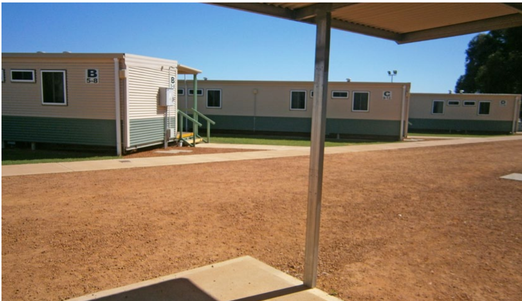
The front view of a Unit 4 accommodation block, showing the verandah where prisoners congregate, and the rear view of the blocks from the front of the unit office.
