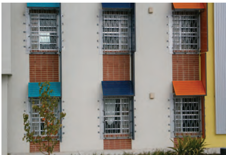
Photo 13: Grilles retrofitted to Urquhart Unit cell windows.
