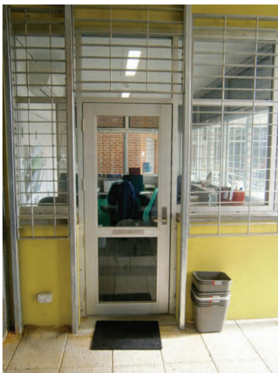
Photo 8: Retrofitted security around unit office windows.
