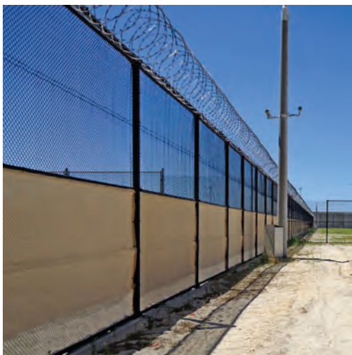
Photo 20: Shadecloth added to perimeter fencing of Hakea Units 11 and 12.
