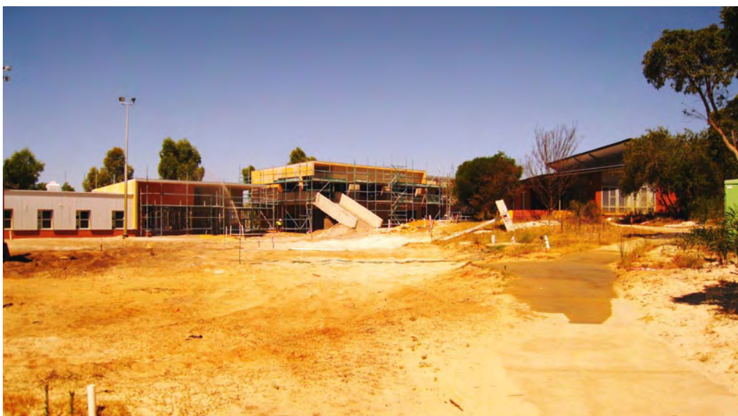
Figure 2: Young women & girls precinct under construction (Jan 2012).
