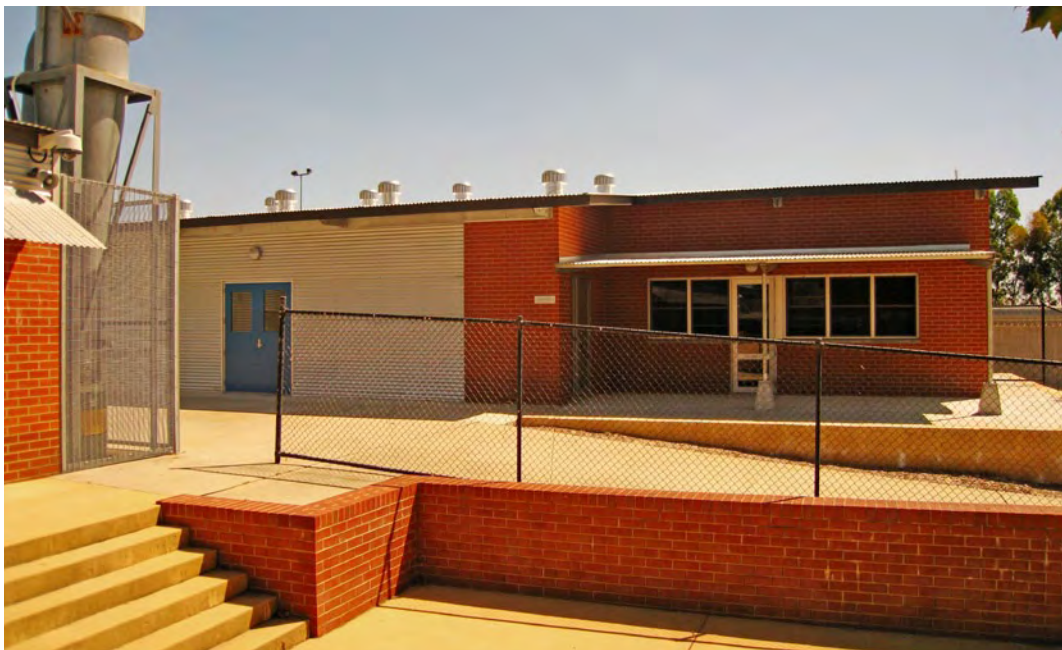
Figure 10: New workshop and training room in the main school area.
