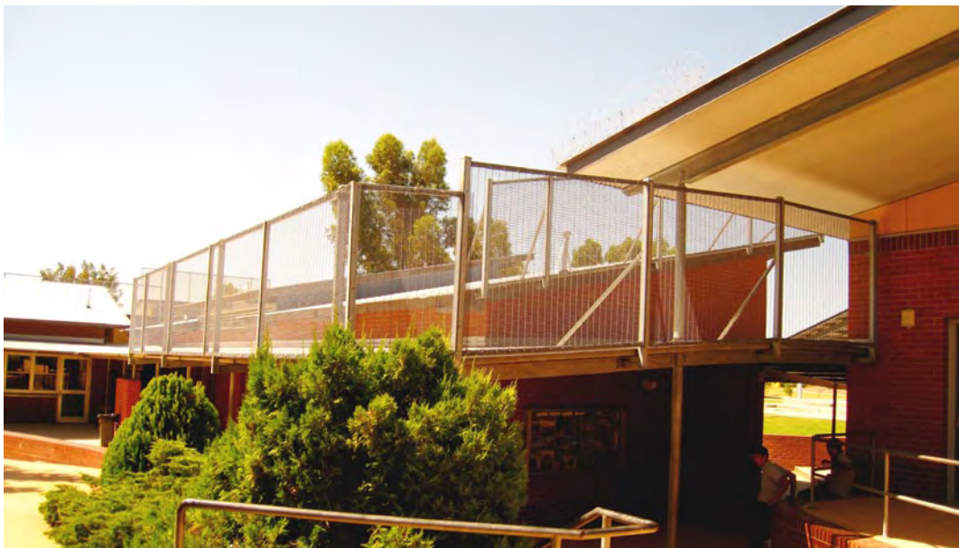
Figure 3: Modifications to reduce roof access by detainees.
