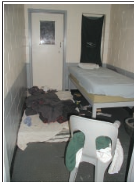
Cell in security section
