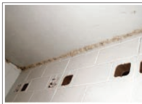
Papier mache moulded into the cracks
