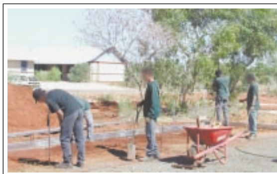
Prisoner students preparing for a concrete pour at the TAFE campus
