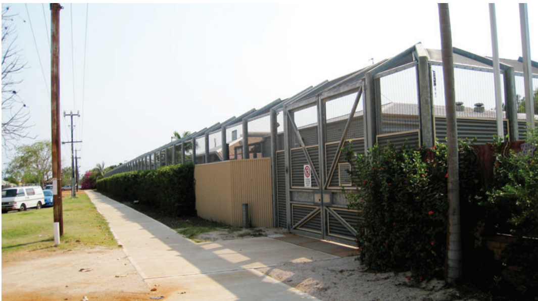
Broome Regional Prison's external fence profile from a street view.
