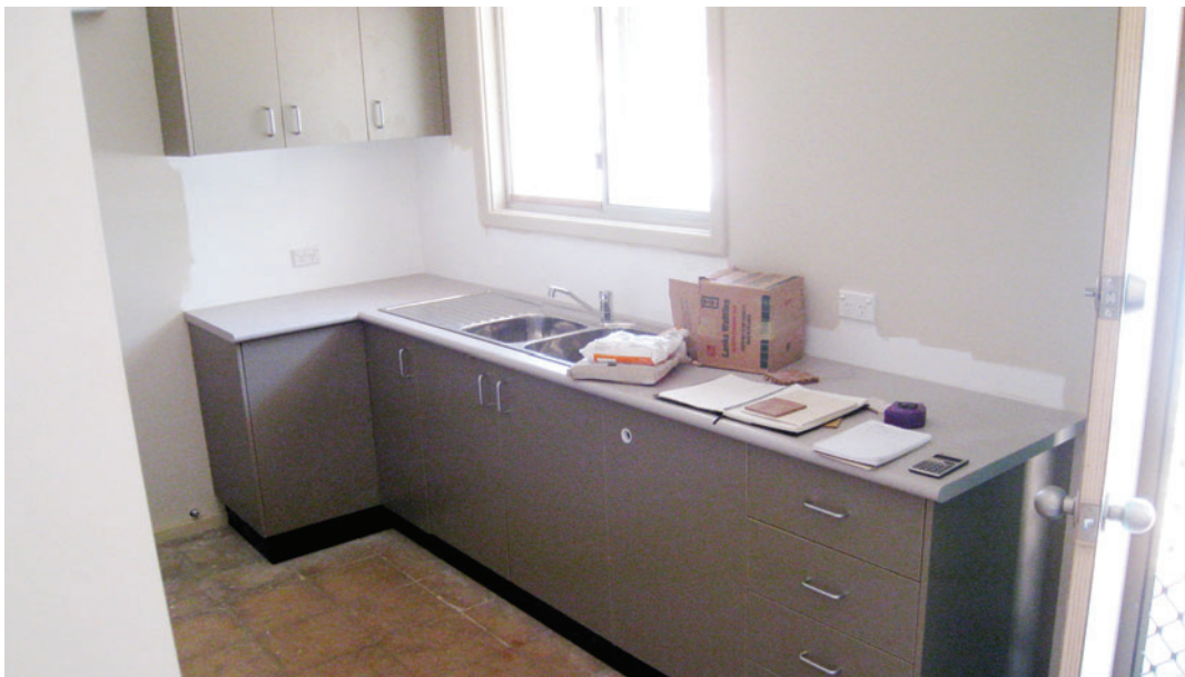
Housing project being undertaken by Broome Regional Prison section 95 prisoners.
