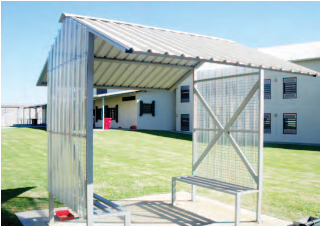
Figure 14: Smoking shelter at Unit 11
