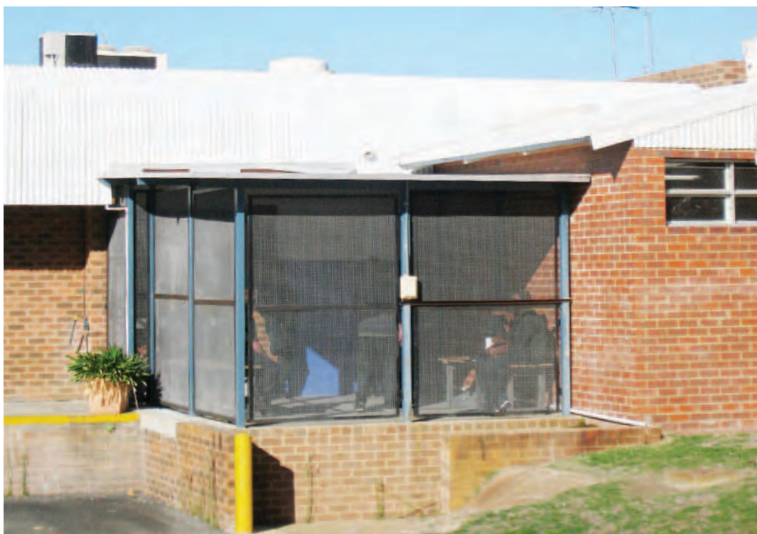
Figure 5: Outdoor caged holding area for smokers at the video-link facility
