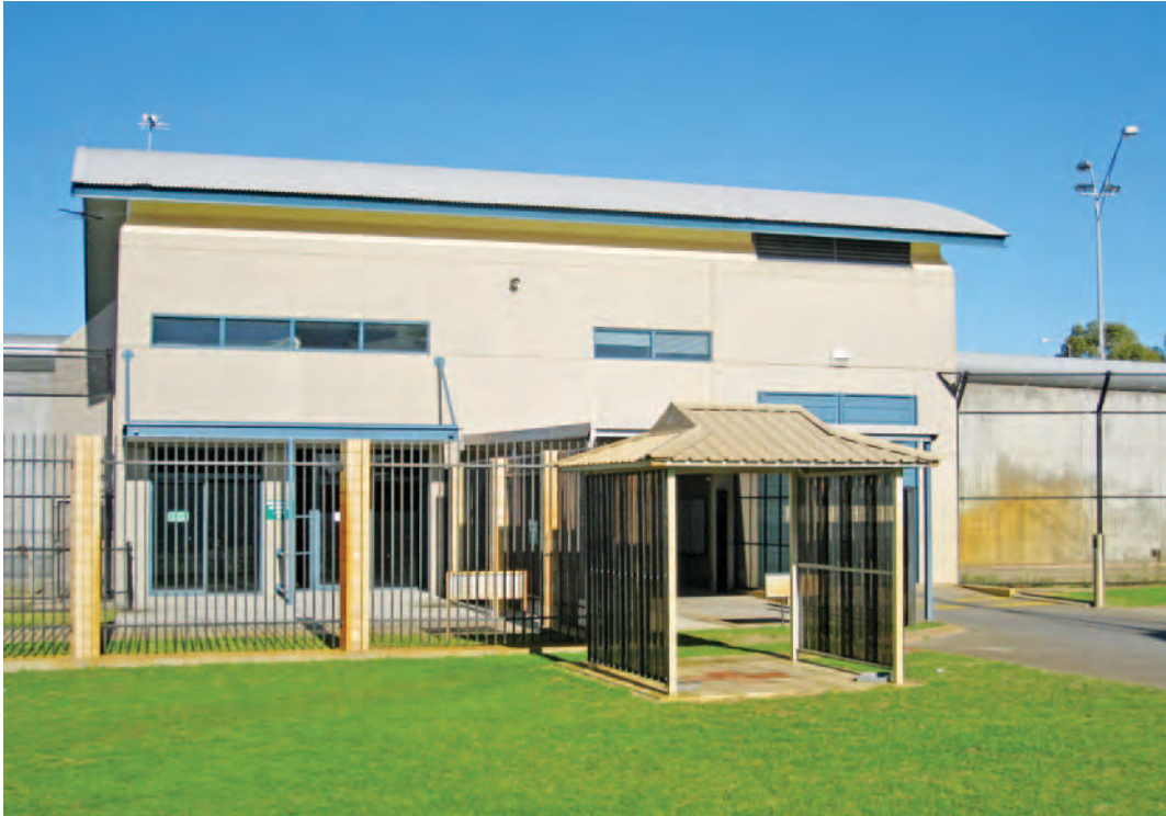
Figure 10: Hakea gatehouse from the inside
