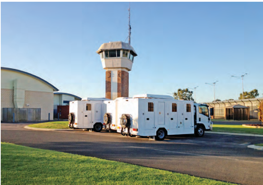
Figure 4: Transports awaiting pickups for morning court runs
