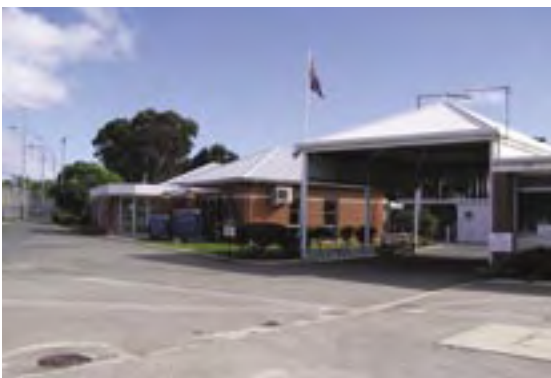
The existing entrance to the prison.
