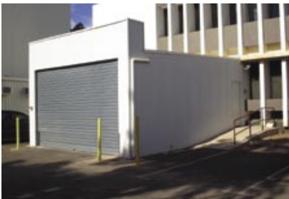
7. New sally port addition outside the Kalgoorlie custody area.
