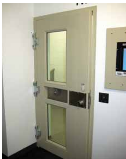
holding rooms 02 at court room levels
