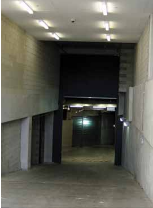
escort vehicle entry to sally port
