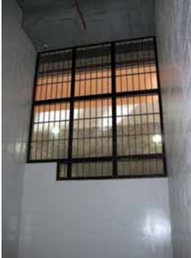
holding courtyard external screen
