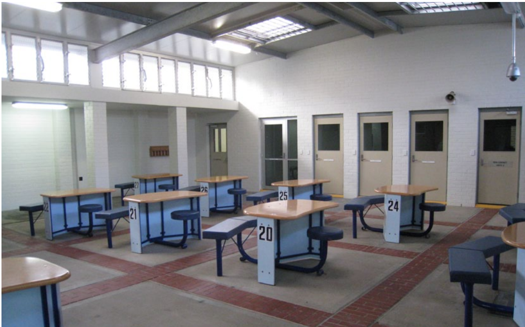
An improved outdoor visits area in response to previous recommendations made by this Office.
