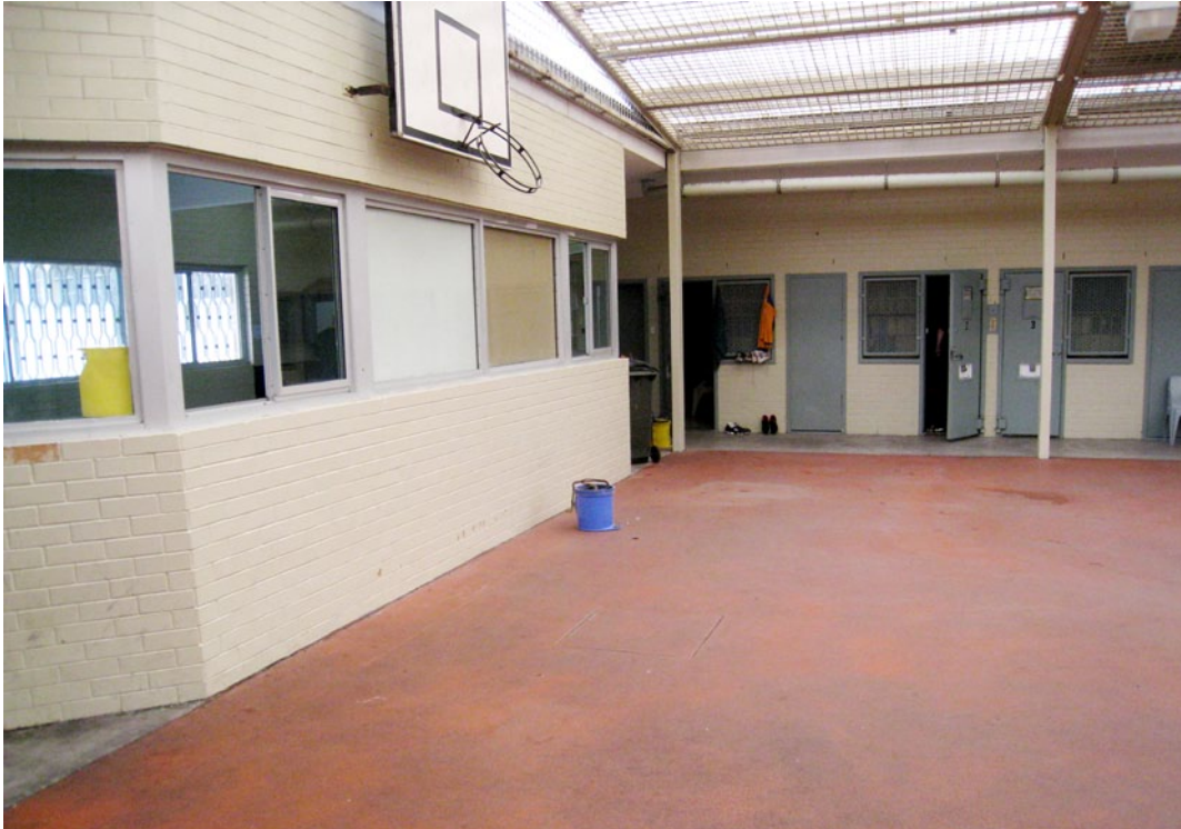
Figure 1: Unit One B Yard
