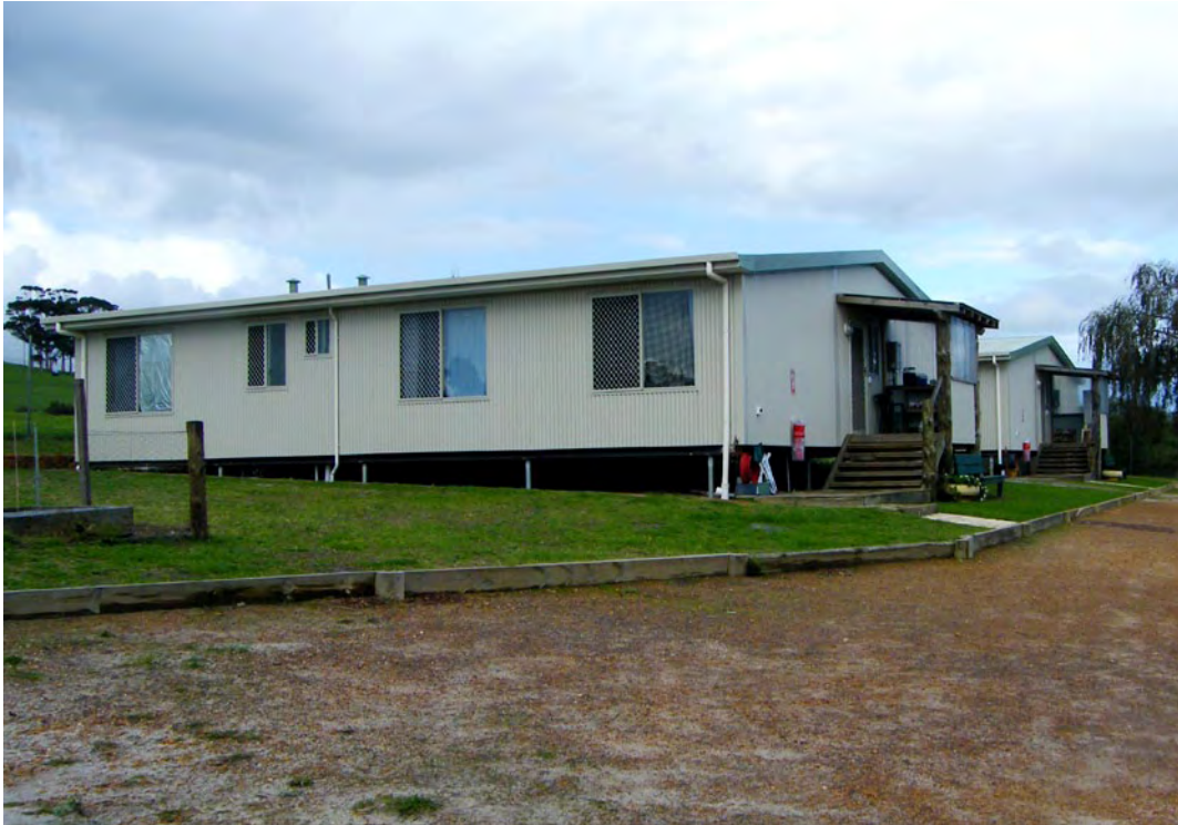
Figure 2: Walpole Work Camp accommodation
