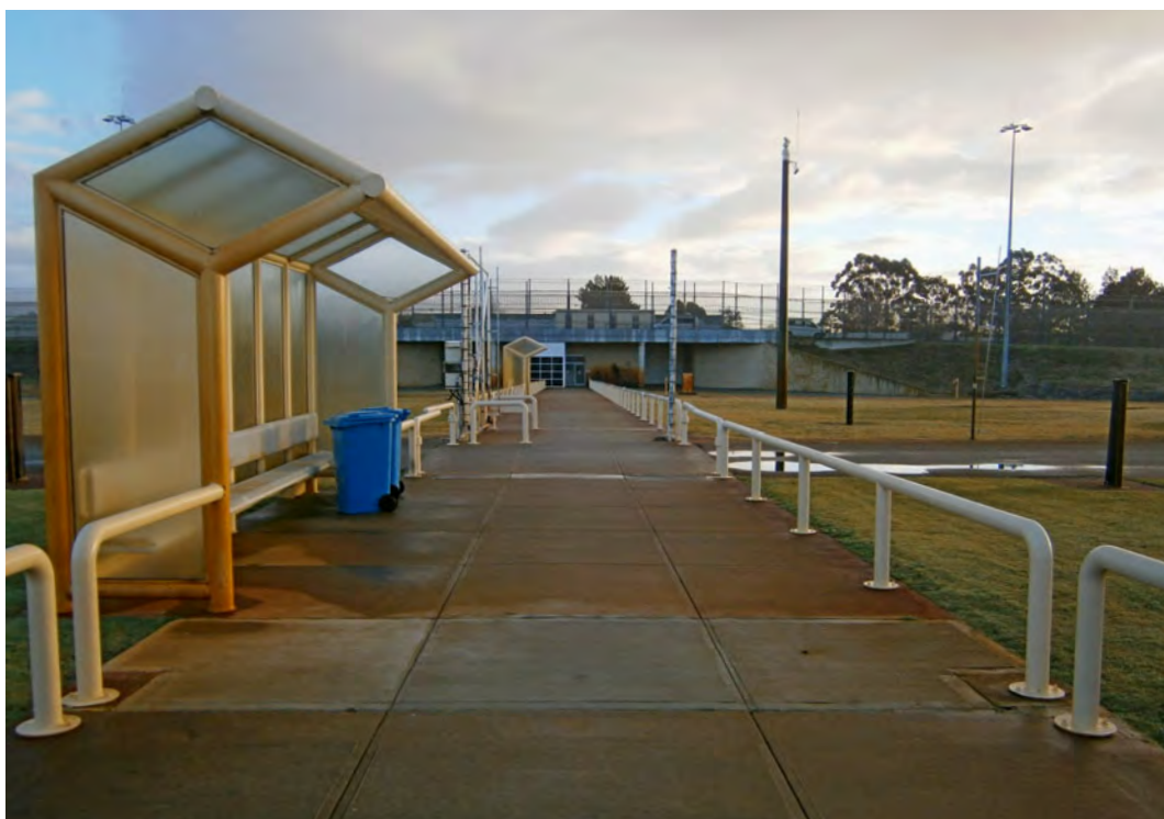
Figure 1: The walkway from the gatehouse into the prison
