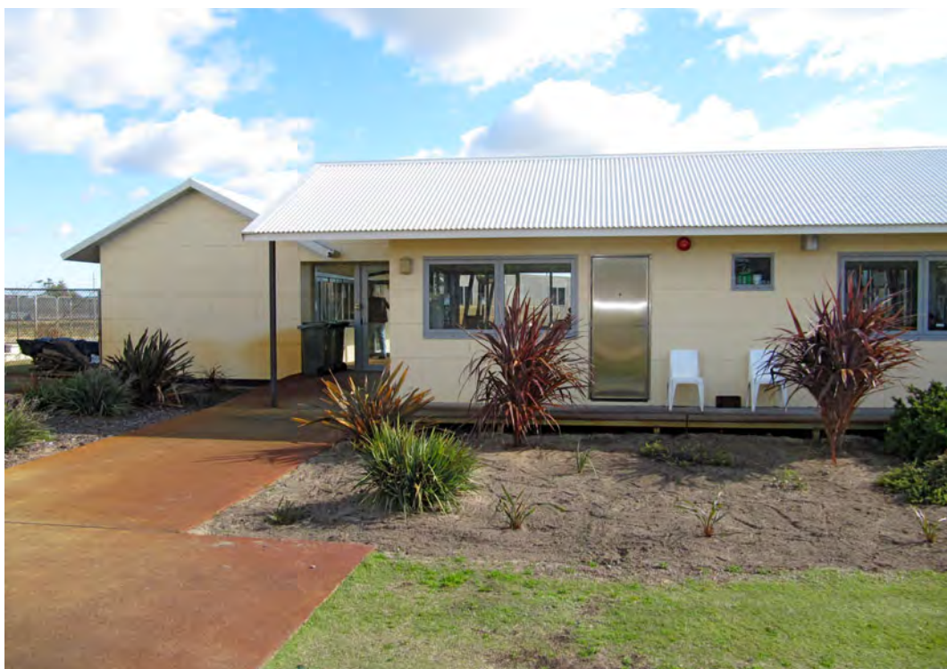
Figure 18: A well-designed facility
