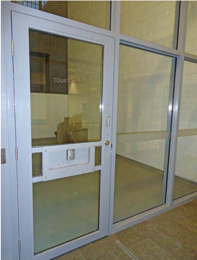
Photo 3: The unused court yards at the District Court Building
