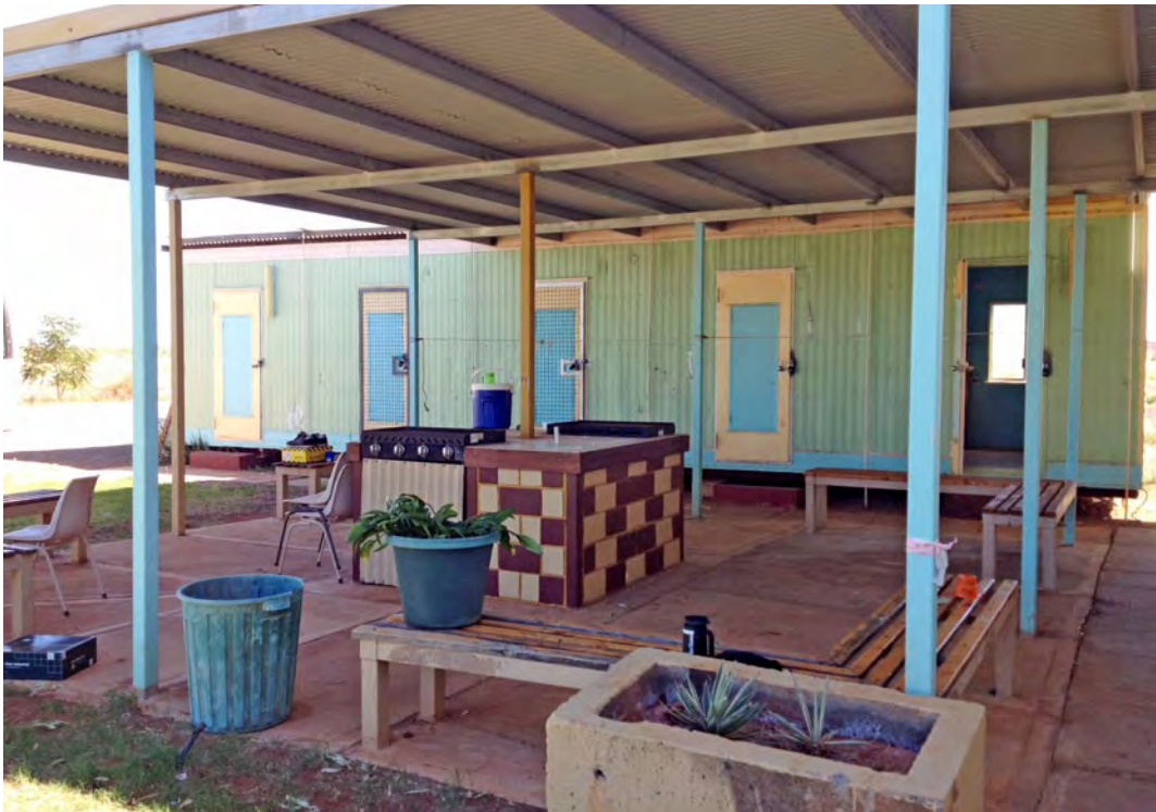
Figure 18: The patio and BBQ at DECCA – one of many construction projects undertaken there.
