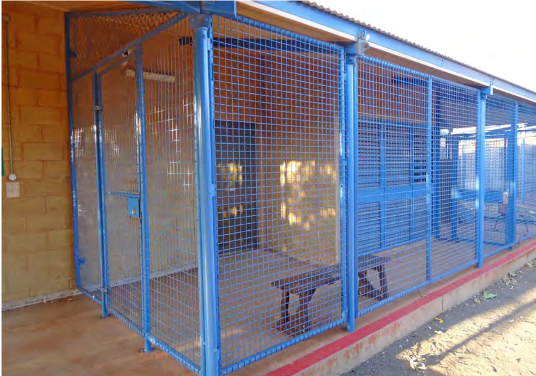
Figure 14: The waiting area adjacent to the Health Centre.
