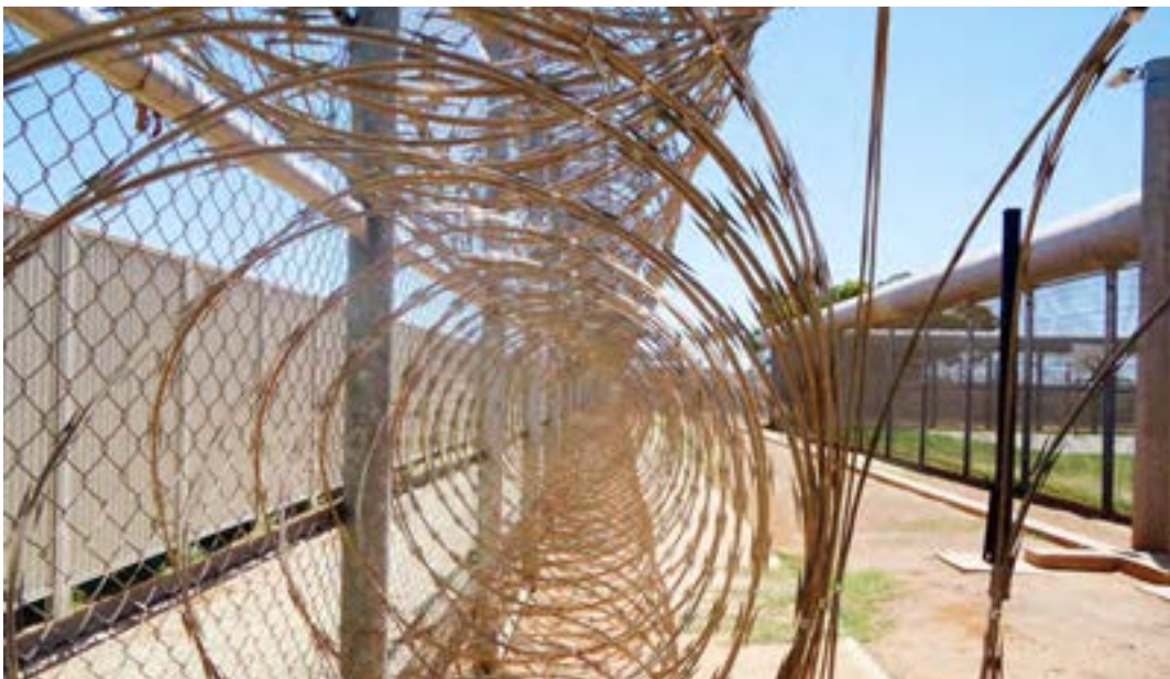
Photo 22: New perimeter fence, razor wire and cowling
