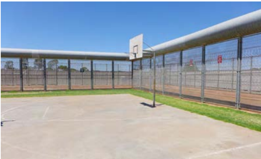
Photo 6: The secure exercise area, with restricted view
