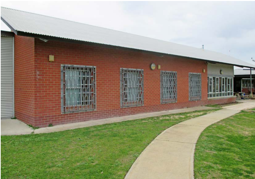
Photo 6 : Cell window grilles on an accommodation unit.
