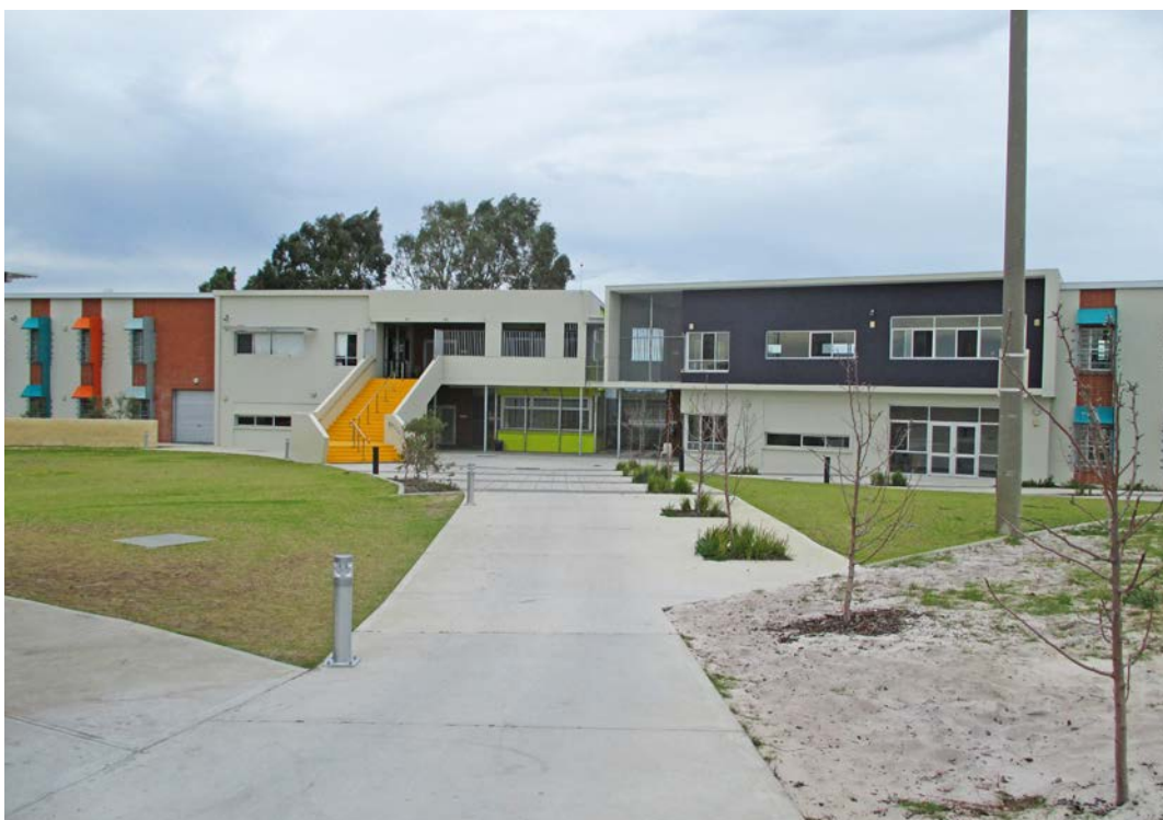
Photo 5 : The construction of the double-storey Urquhart Unit was a departure from the earlier design philosophy of domestic scale.
