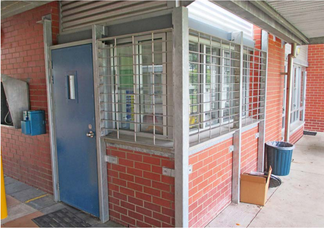
Photo 7 : A unit office with retrofitted fortification.
