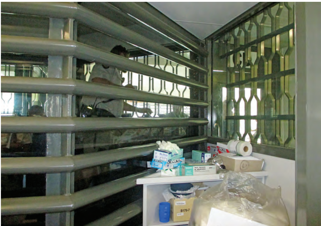
Photo 4: The heavy grills on the Unit 3 control room.
