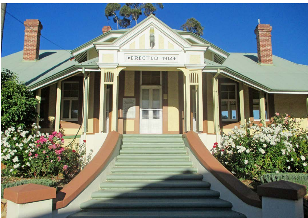
Photo 1: The administration building – a piece of history.
