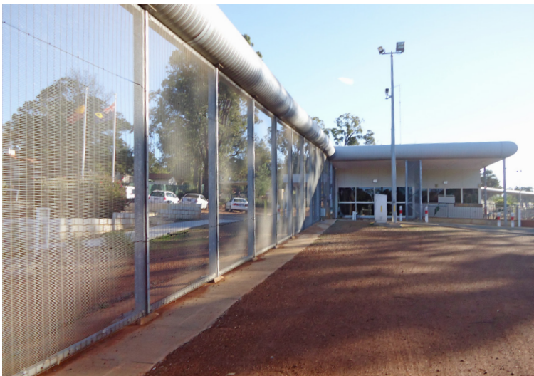
Photo 7: Wooroloo's perimeter fence and gatehouse.
