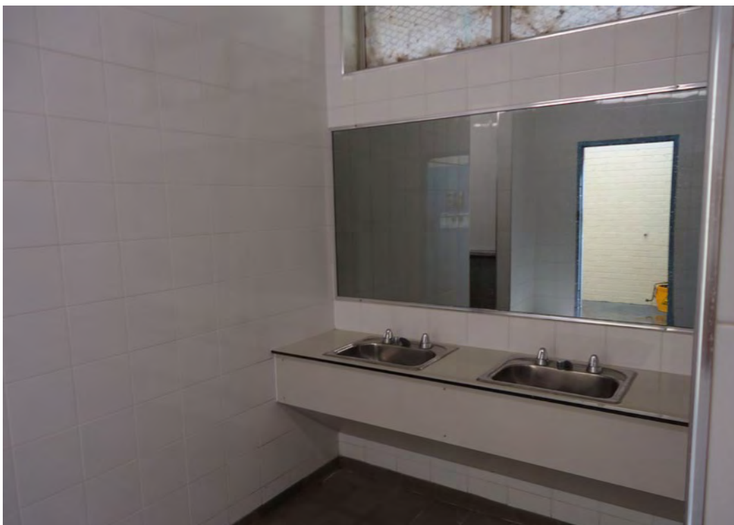
Figure 7: The newly refurbished bathrooms in Units 2 and 3 were of a high standard.
