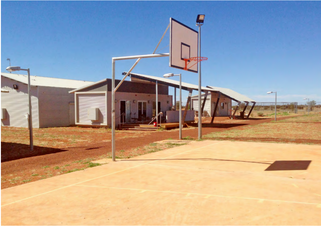
Photo 12 : Basketball court and service facilities at Warburton
