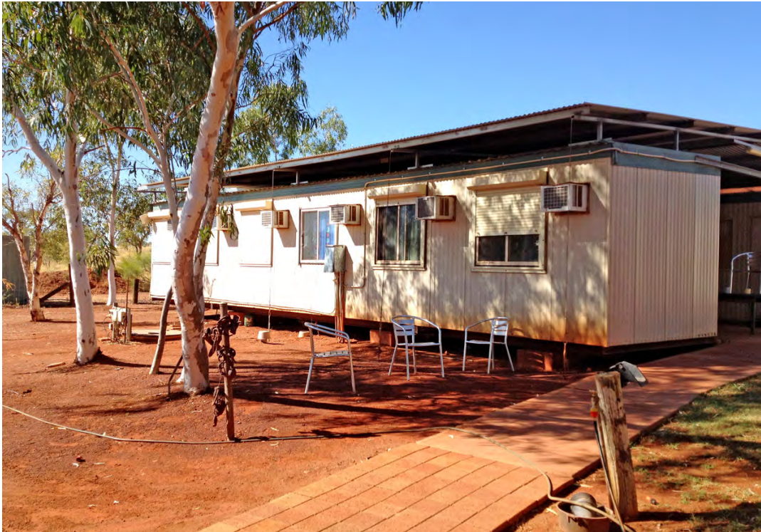
Photo 4 : Millstream prisoner accommodation
