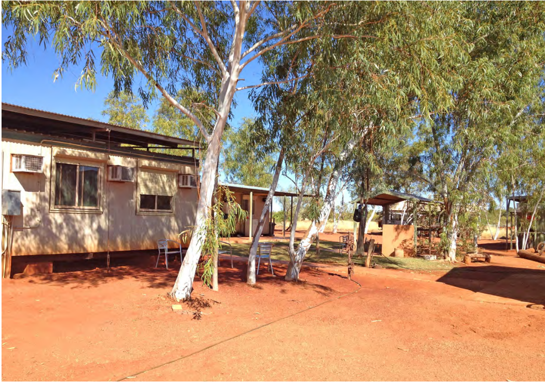
Photo 5 : Millstream prisoner accommodation
