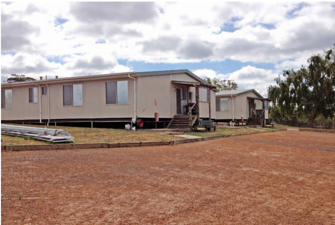
Photo 1 : Walpole prisoner accommodation units
