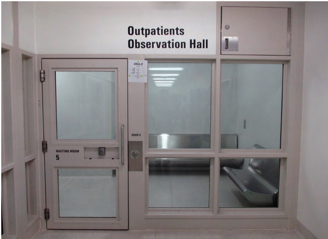
Figure 8: The new secure facility at Fiona Stanley Hospital
