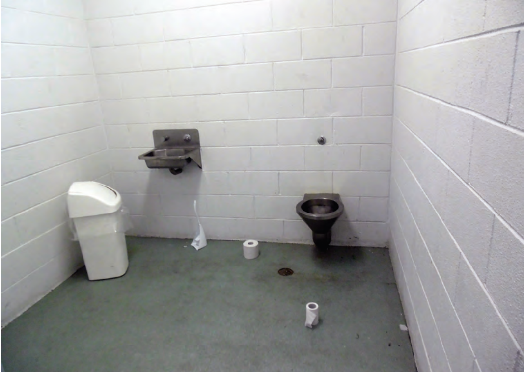
Figure 2: This toilet was sometimes used as a holding area for protection prisoners
