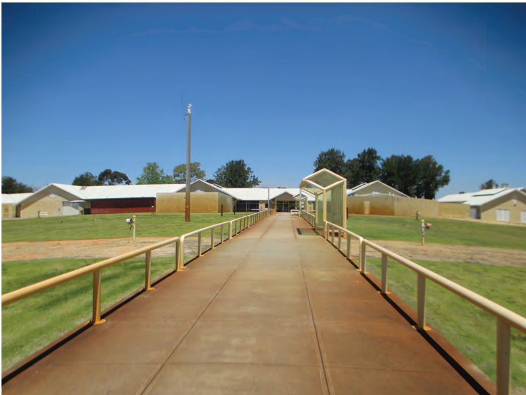
Figure 1: The entry path to Casuarina Prison, leading to the administration building and visits centre
