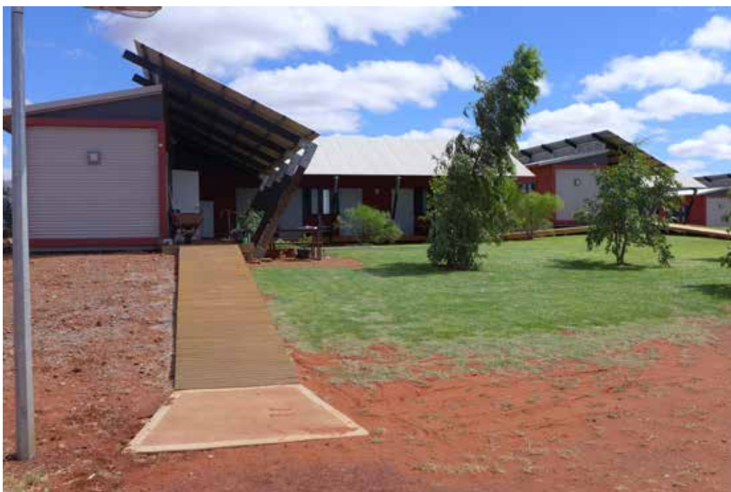
Figure 18: Warburton Work Camp accommodation
