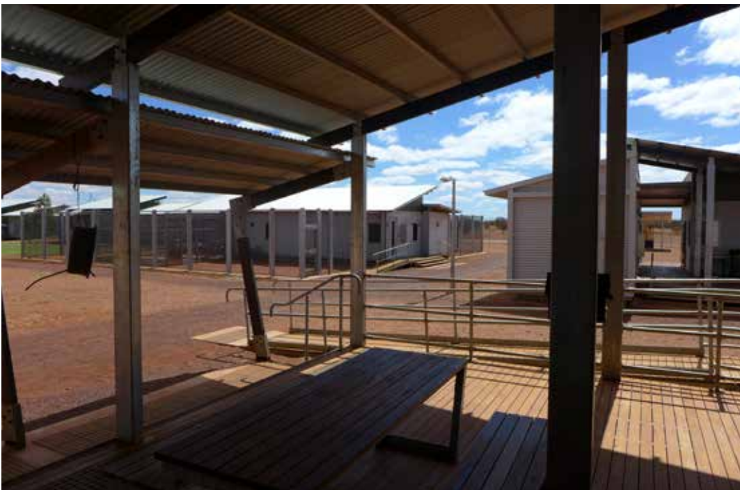
Figure 19: Warburton Work Camp secure facility
