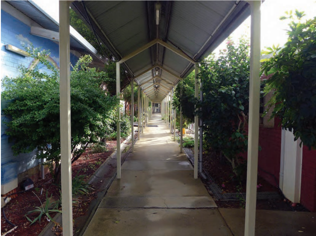
Photo 1: Walkway behind Unit 1
