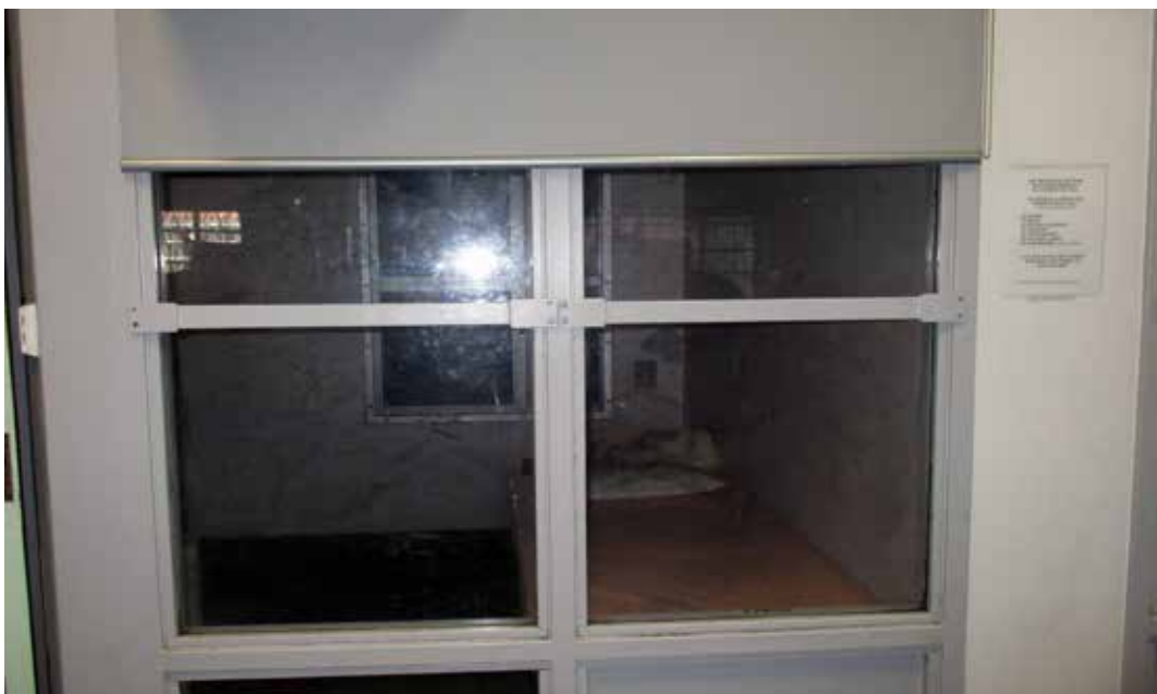
Photo 9 and 10: The interior and exterior of an observation cell
