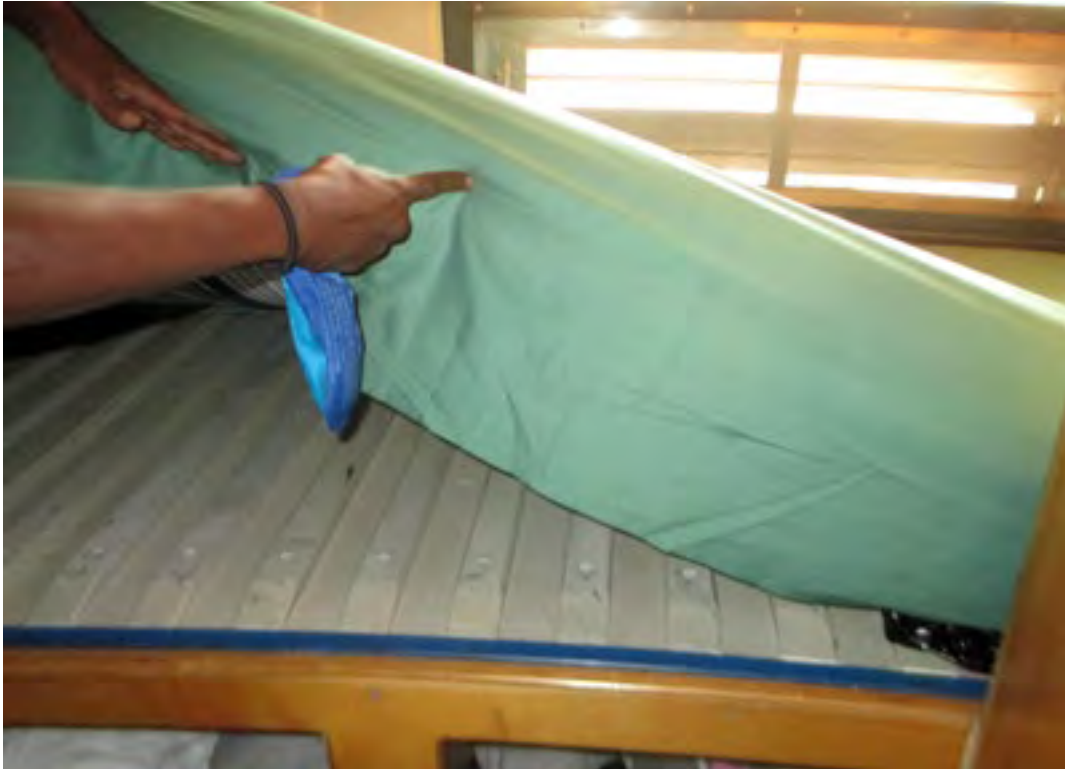
Photo 7-10: Raised slats on bed bases could be felt through the thin mattresses
