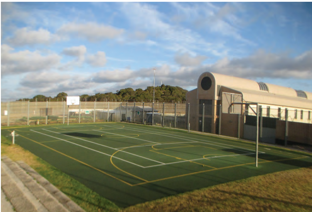
Photo 14: Looking across Unit 4's fine basketball court towards Unit 3
