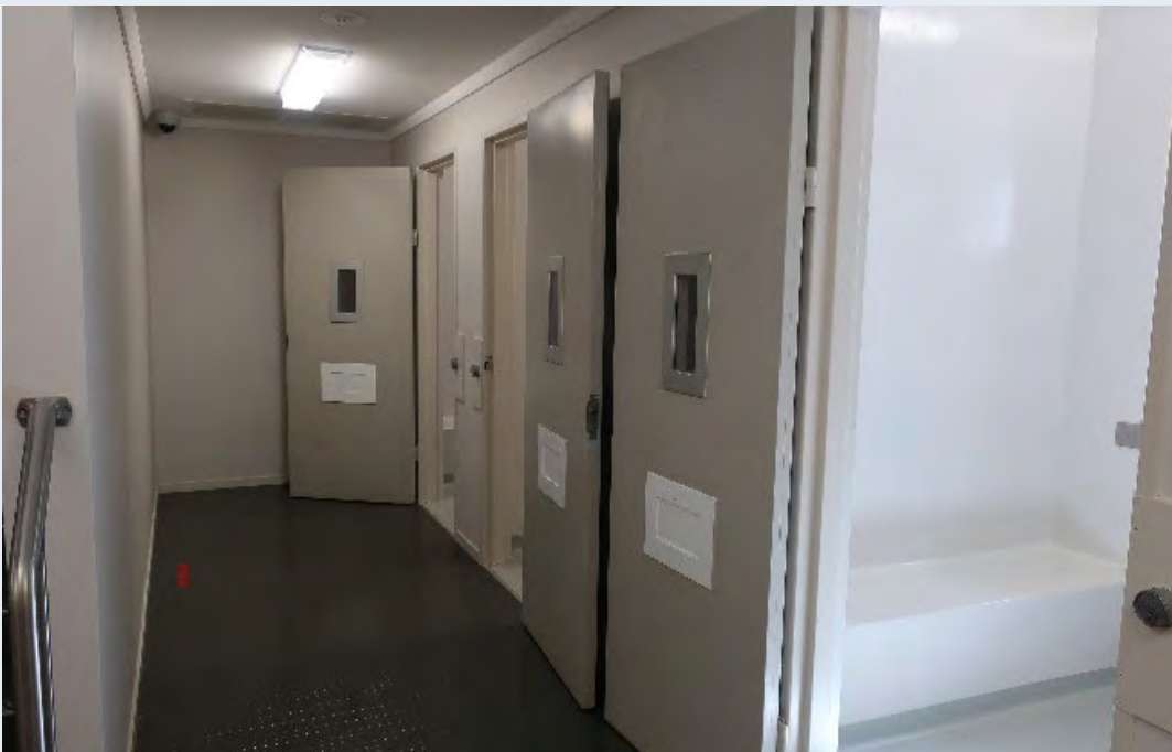
Photo 38. Kununurra Court police lock-up
