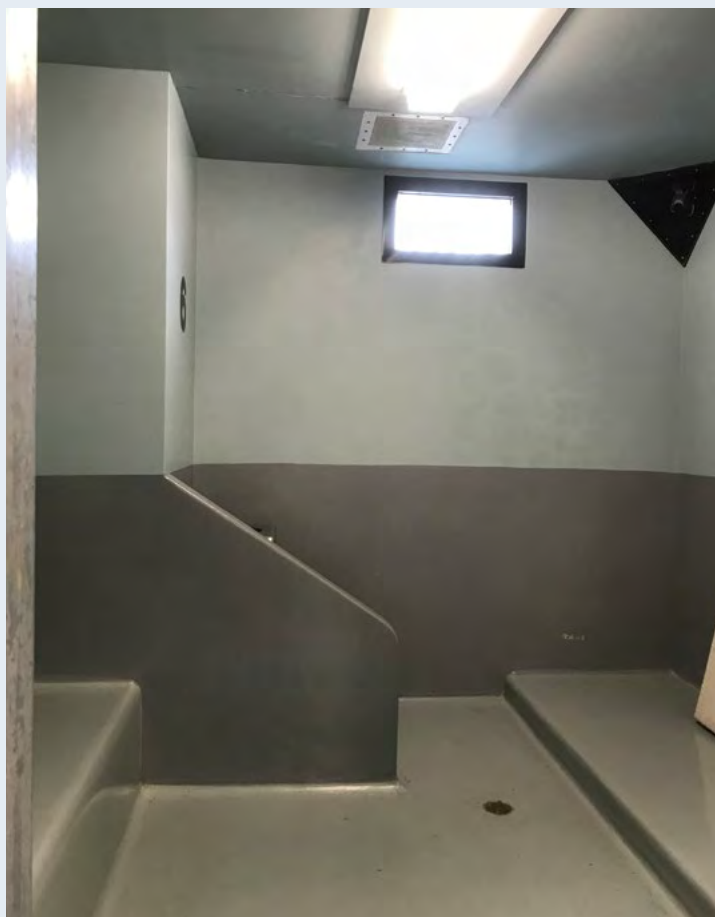
Photo 25. Albany Court holding cell
