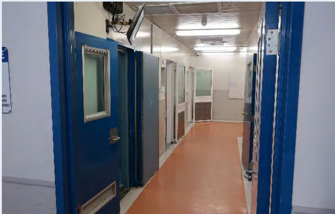
Photo 34. Geraldton Court custody centre
