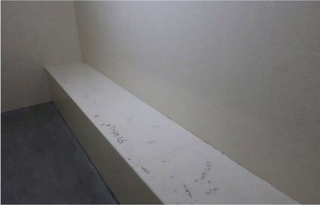
Photo 29. Bunbury Court holding cell
