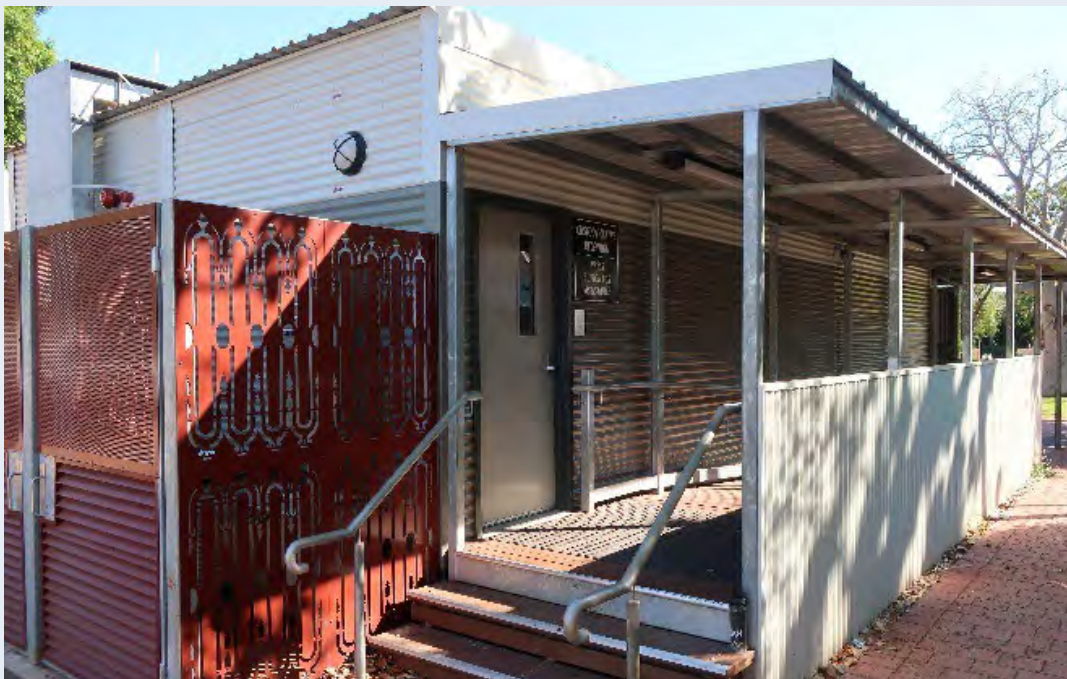
Photo 28. New Broome Court custody building
