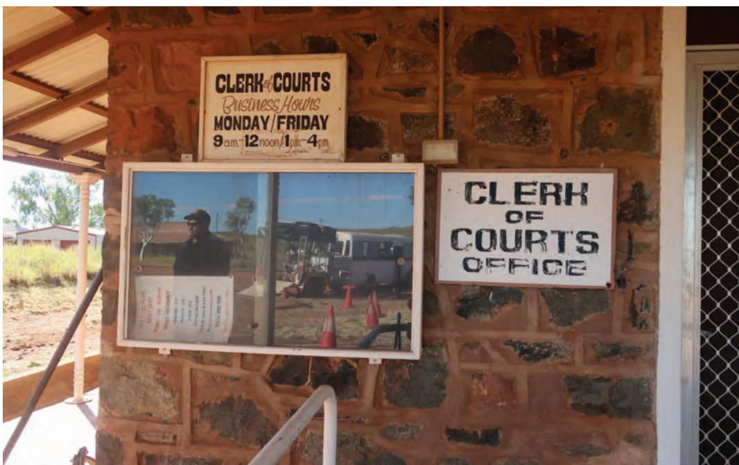
Photo 15: External work at old Roebourne Courthouse.
