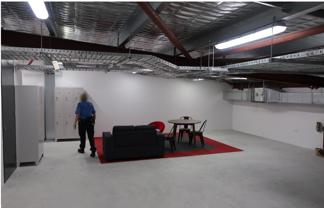
Photo 2: Staff amenities at the gatehouse.
