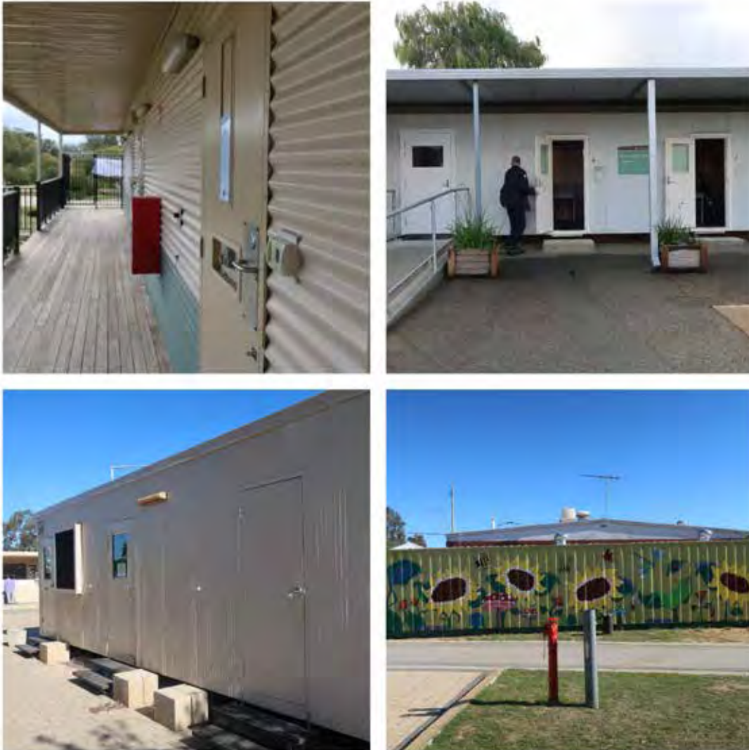
Photo 2: Dongas and sea container used for prisoner accommodation, official visits, staff offices and reception storage (among other purposes)
