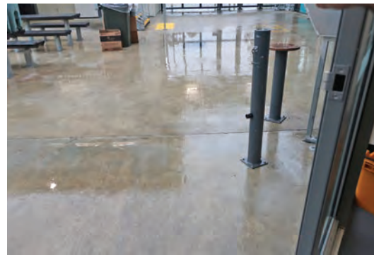
Photo 11: Unit 6 roof line did not have gutters Photo 12: Unit 6 lacks adequate drainage
