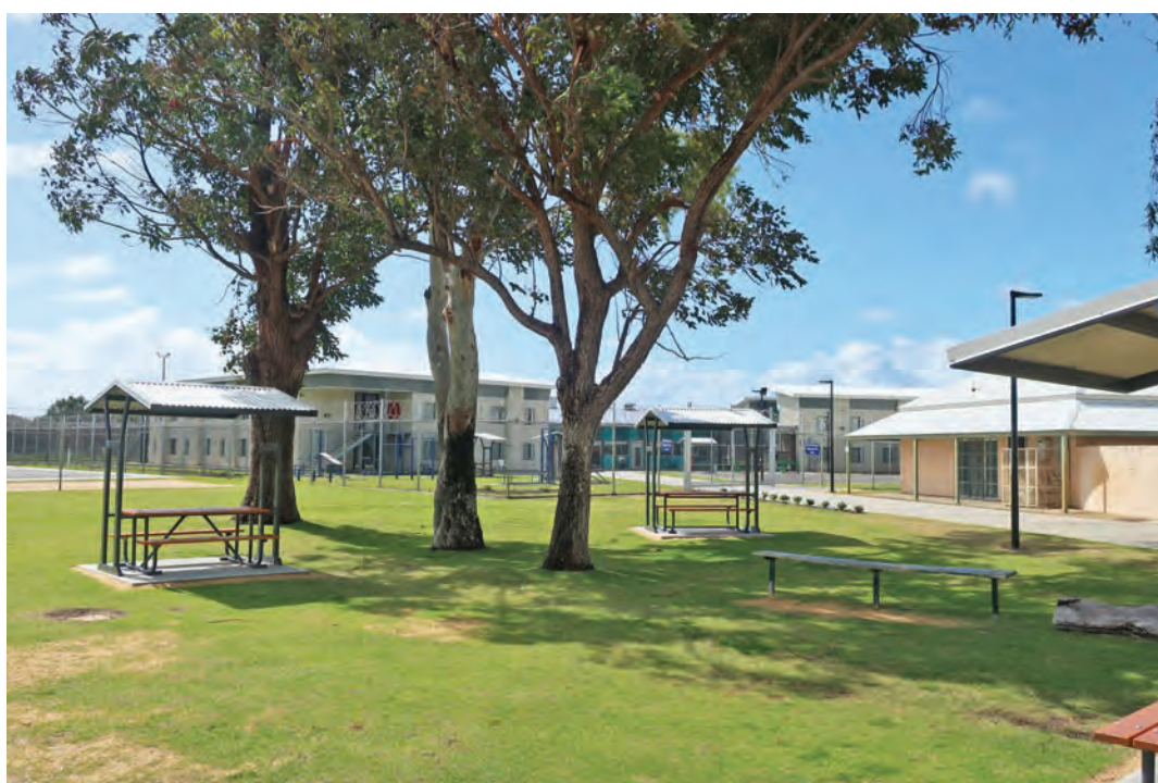
Photo 3: The new Unit 6
