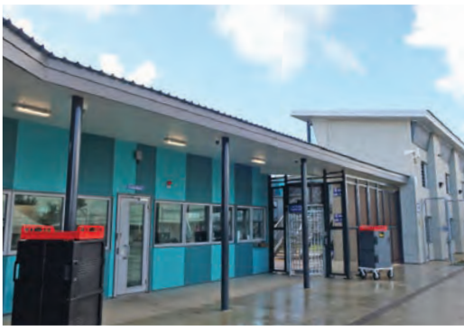
Photo 11: Unit 6 roof line did not have gutters Photo 12: Unit 6 lacks adequate drainage
