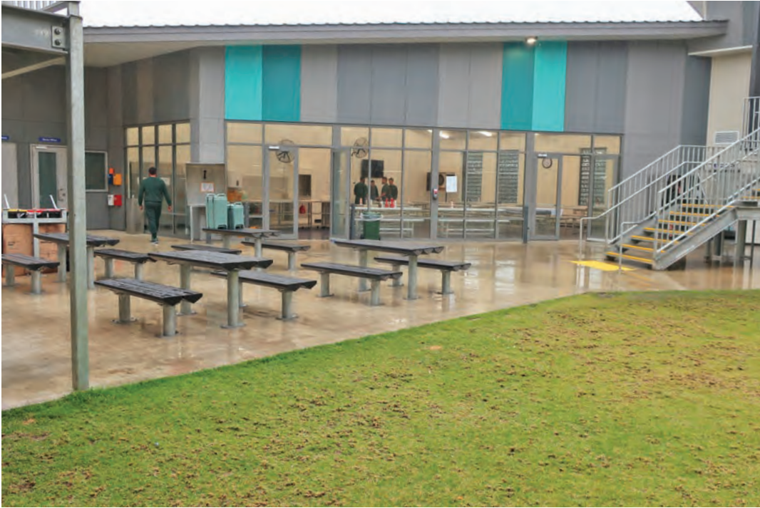
Photo 10: Unit 6 exposed to the weather
