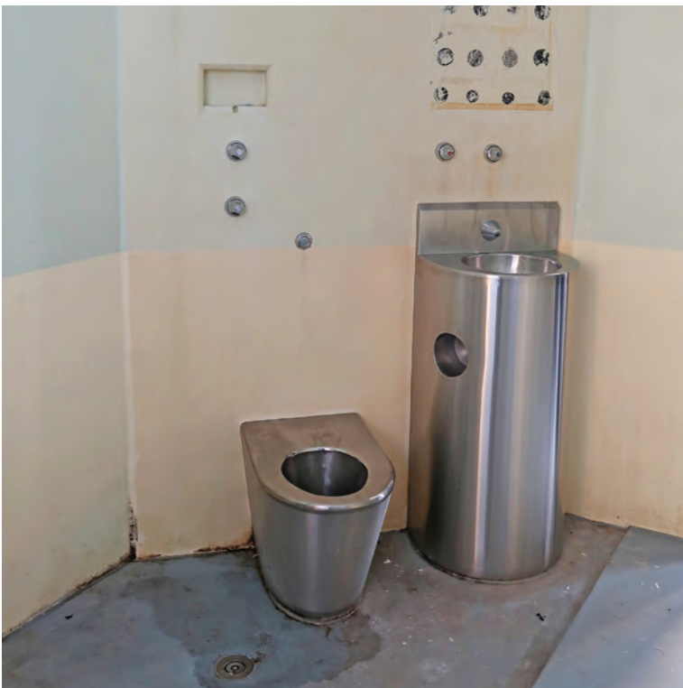
Photo 13: The facilities in one of the Crisis Care cells
