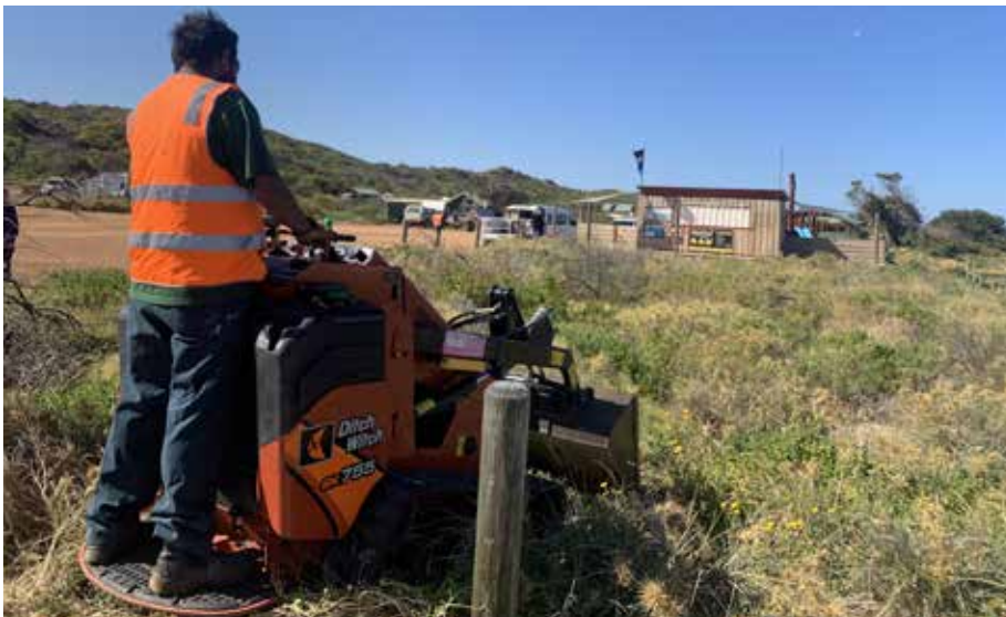
Photo 17: Men working on dune restoration
