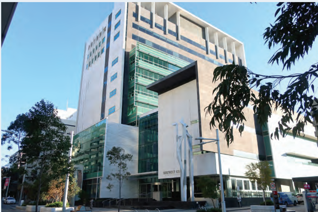
Photo 8: District Court Building: commissioned 2008
