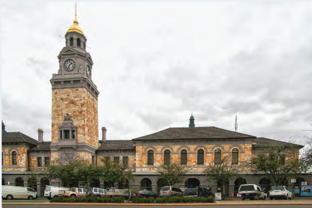
Photo 9: Kalgoorlie Courthouse: commissioned 2013, built 1899
