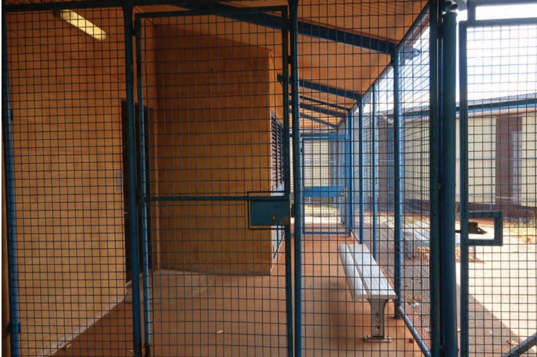
Photo 15: Waiting room cage
