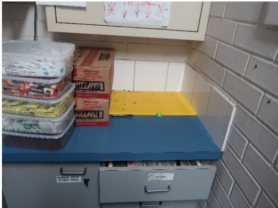
Photo 3 Rat faeces on a unit office cutting board
