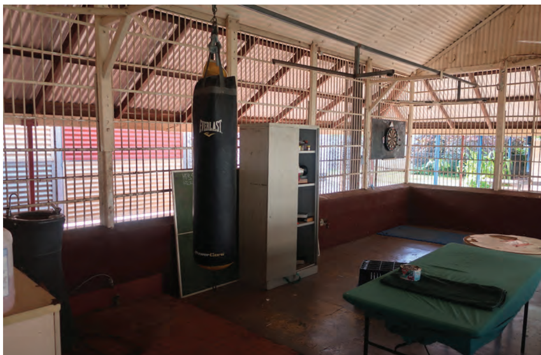
Photo 8. The old “Bull Pen” was dilapidated
